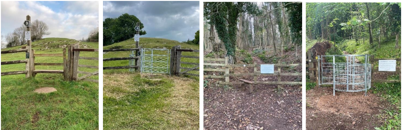
Figure 14 Before and after shots of stile replacements with kissing gates
